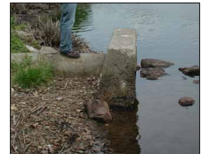
Fig. 1.3 Increased stormwater resulting in riverbank erosion
