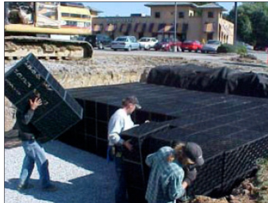
Underground infiltration chamber. Photo source: Rainstay
