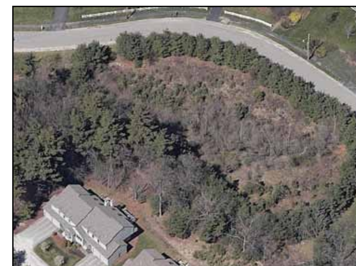
Aerial of existing BMP
