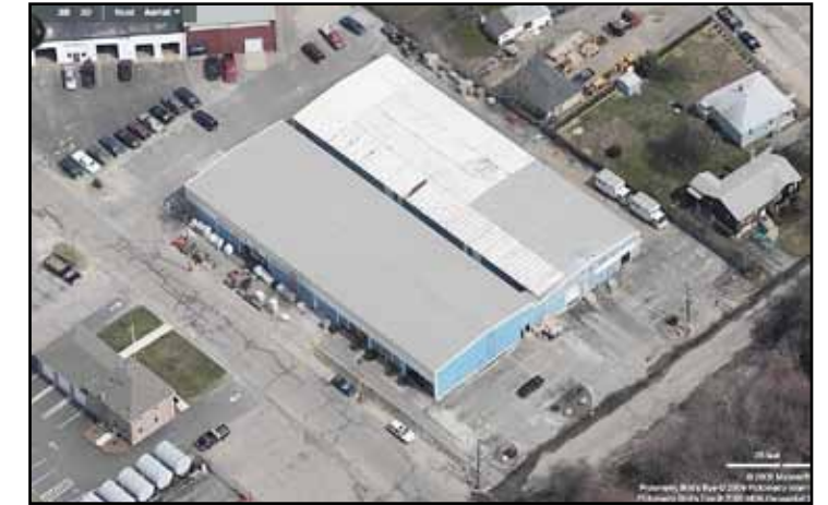
Aerial of hardware store site
