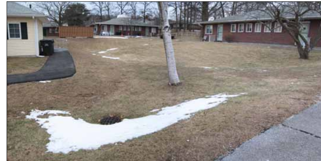
BEFORE: Photo of existing catch basin in existing courtyard.
