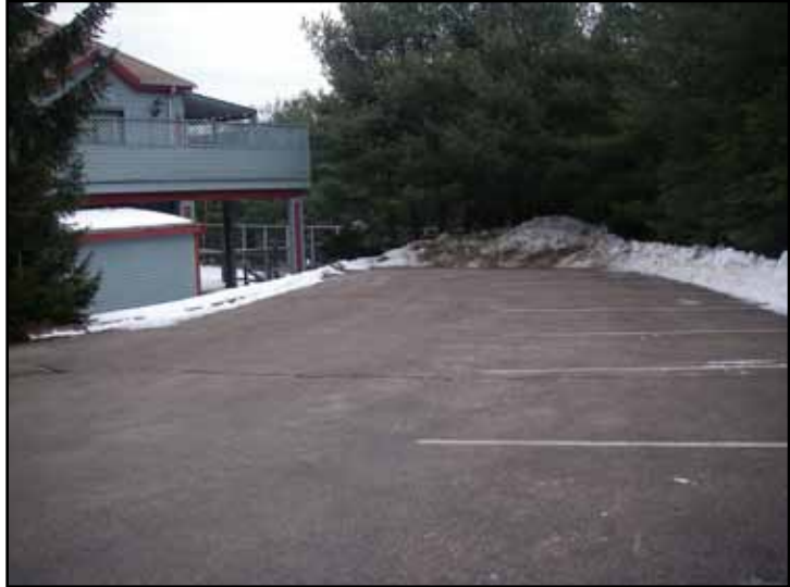
End of parking lot on southeast side of the building
