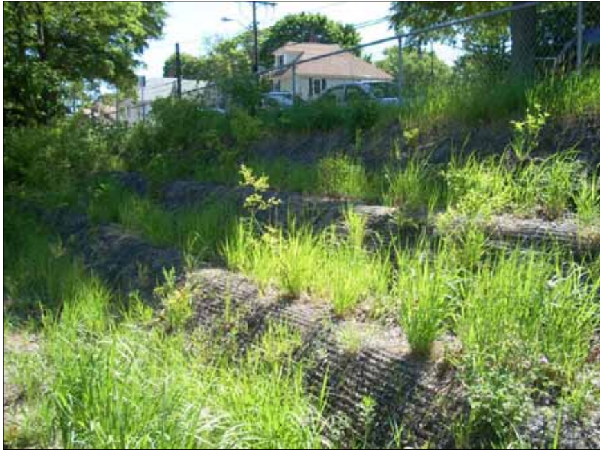
Terraced infiltration basin. Photo source: Horsley Witten Group
