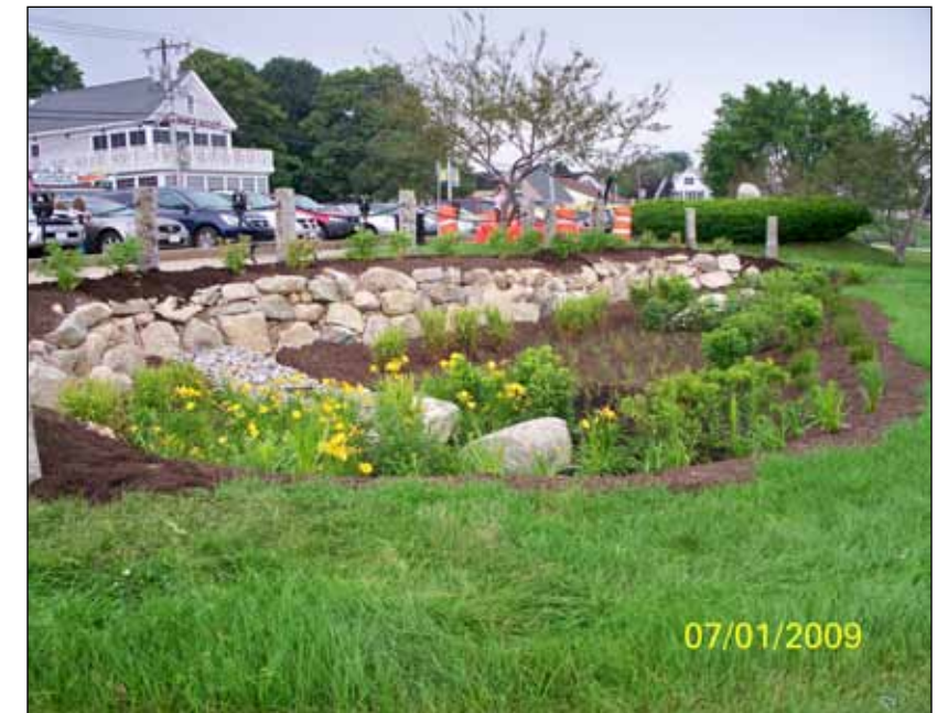
Infiltration basin. Photo source: Horsley Witten Group
