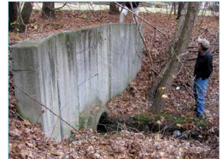
Project team member observing existing drainage pattern.
