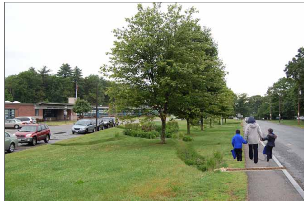
AFTER: Visualization of proposed trench, swale, and bioretention.
