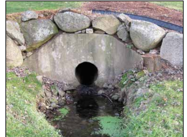
Outflow pipe from Chilmark Road into existing pond
