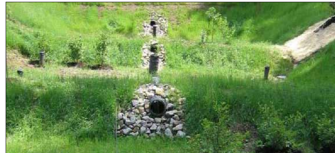
Gravel wetland in use at the University of New Hampshire Stormwater Center.
