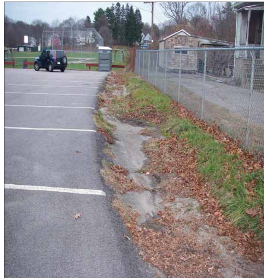
BEFORE: Photo of existing concrete swale on western edge of small parking lot.
