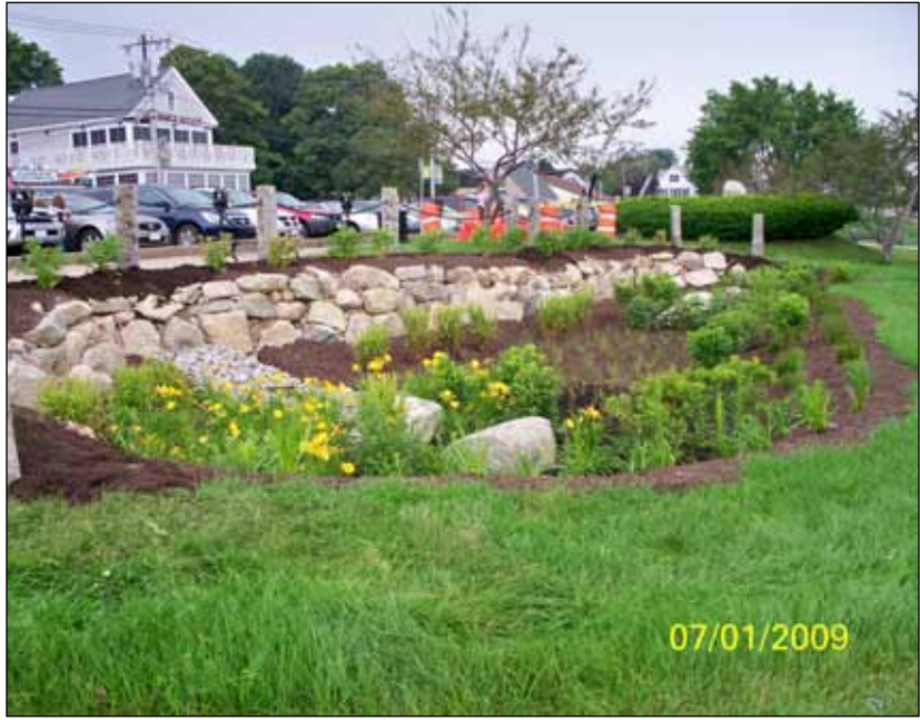
Infiltration basin. Photo source: Horsley Witten Group
